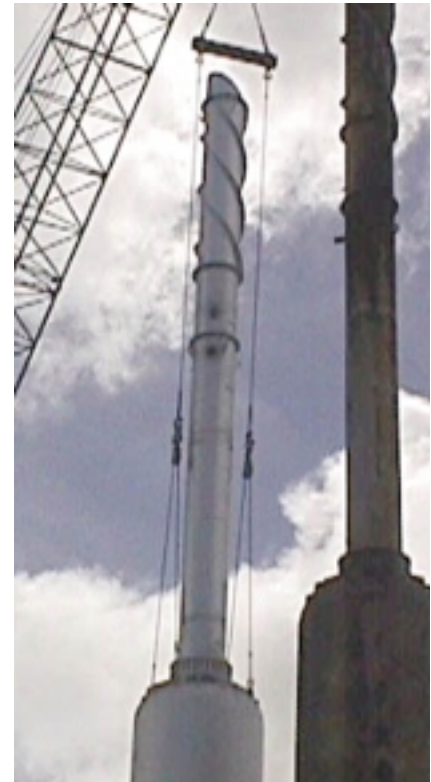
The new silencers and stacks being installed in Guam.
