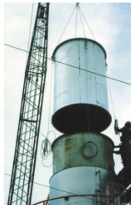
Installation of the Universal Silencer 86-inch-diameter cylindrical silencer with parallel baffles at the General Motors plant in Janesville, WI. Universal Silencer offers a wide range of standard products for a variety of fan applications.
