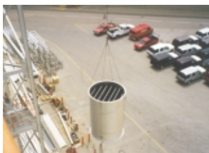
Installation of the Universal Silencer 86-inch-diameter cylindrical silencer with parallel baffles at the General Motors plant in Janesville, WI. Universal Silencer offers a wide range of standard products for a variety of fan applications.
